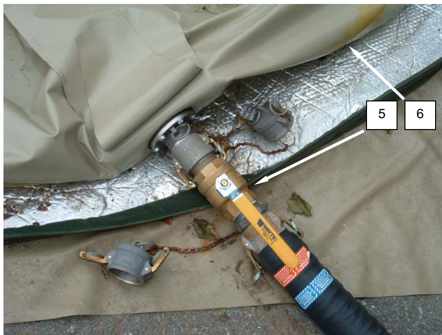
Figure 3. Waste Tank Overflows.
