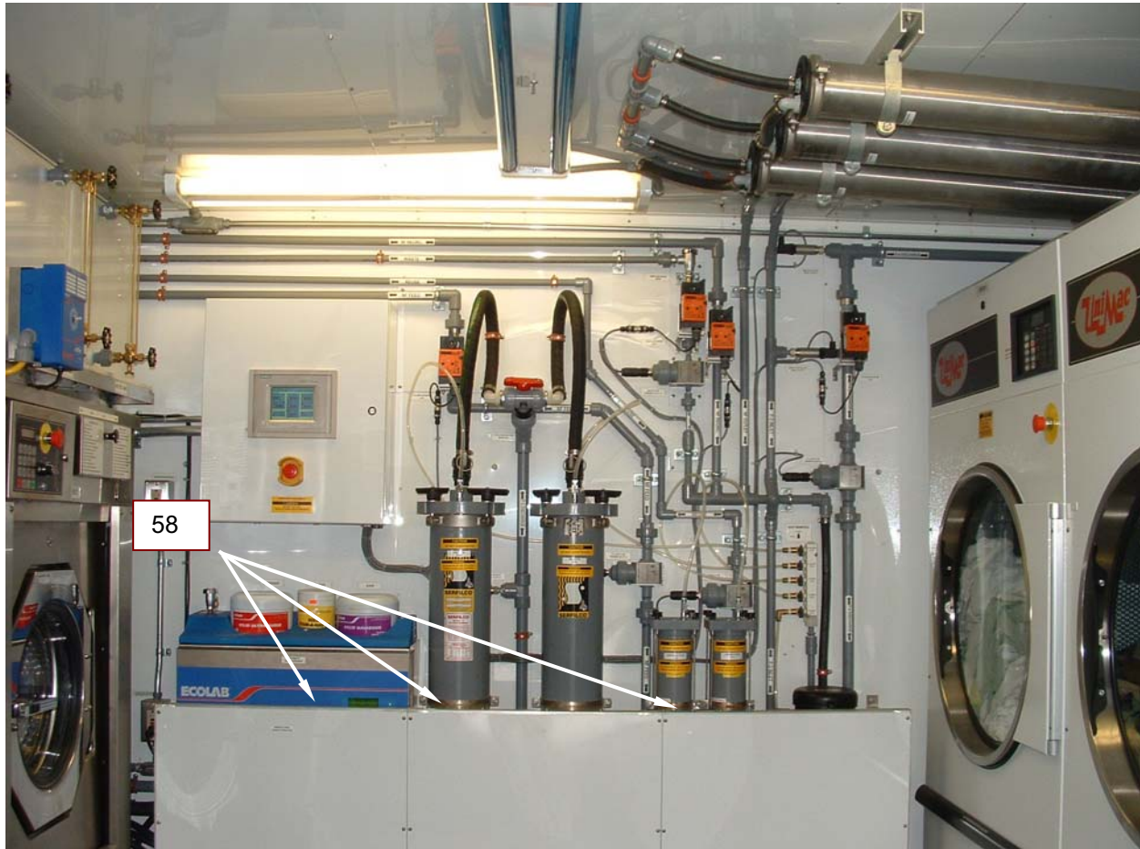
Figure 18. Prepare Filtration System for Use.
