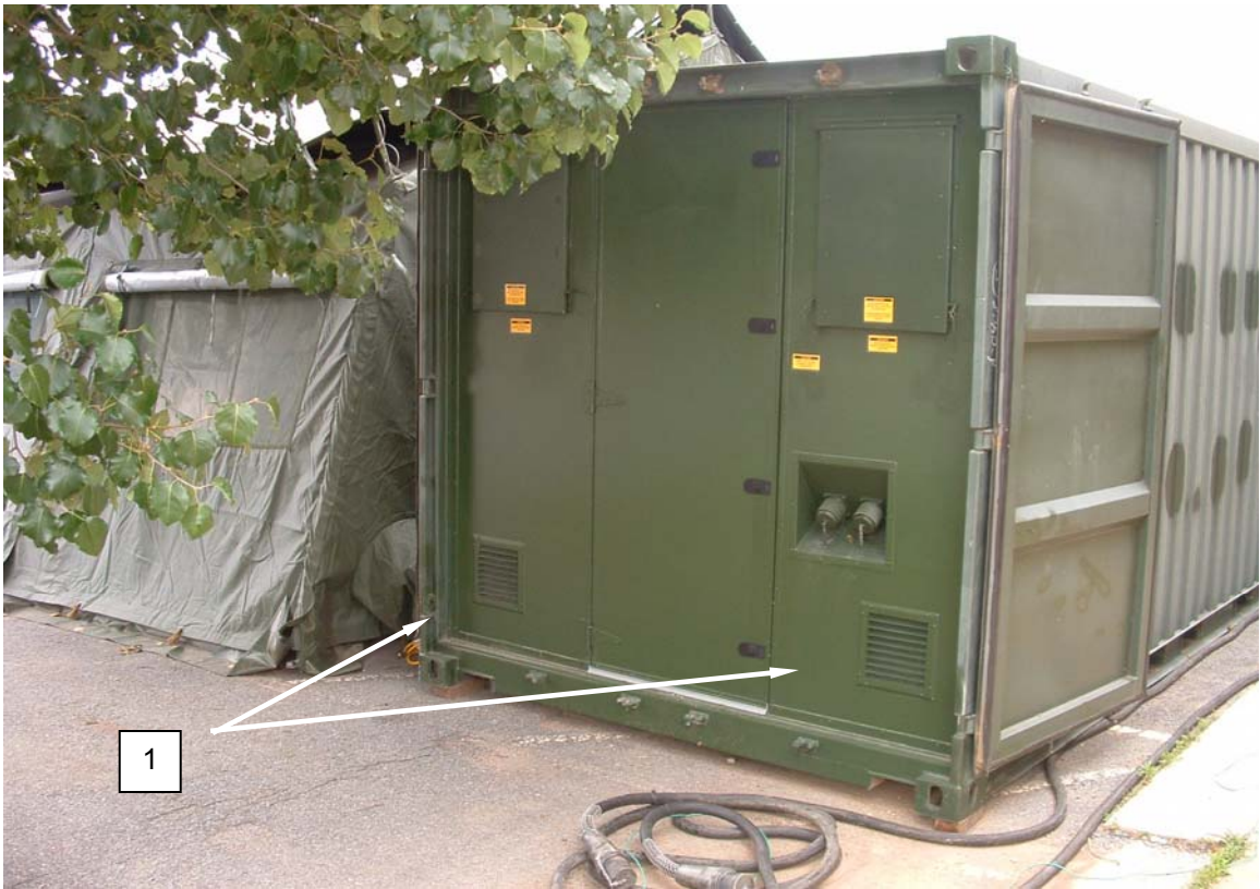
Figure 7. Water in Dryer or Dryer leaking Water.
