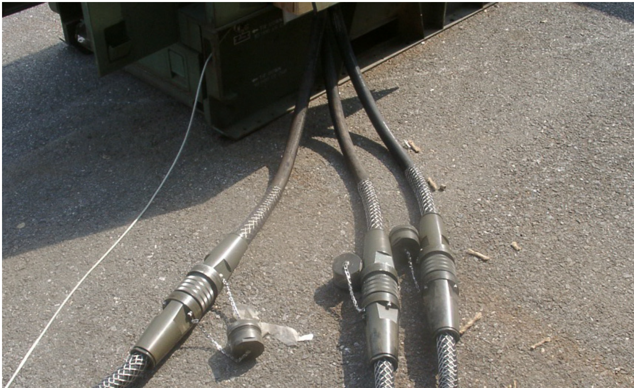
Figure 10. Connect 100 A Pigtail Cables to Generator.
