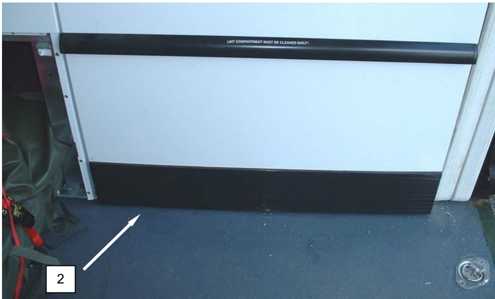
Figure 23. Install Lint Compartment Door on Dryer #2.
