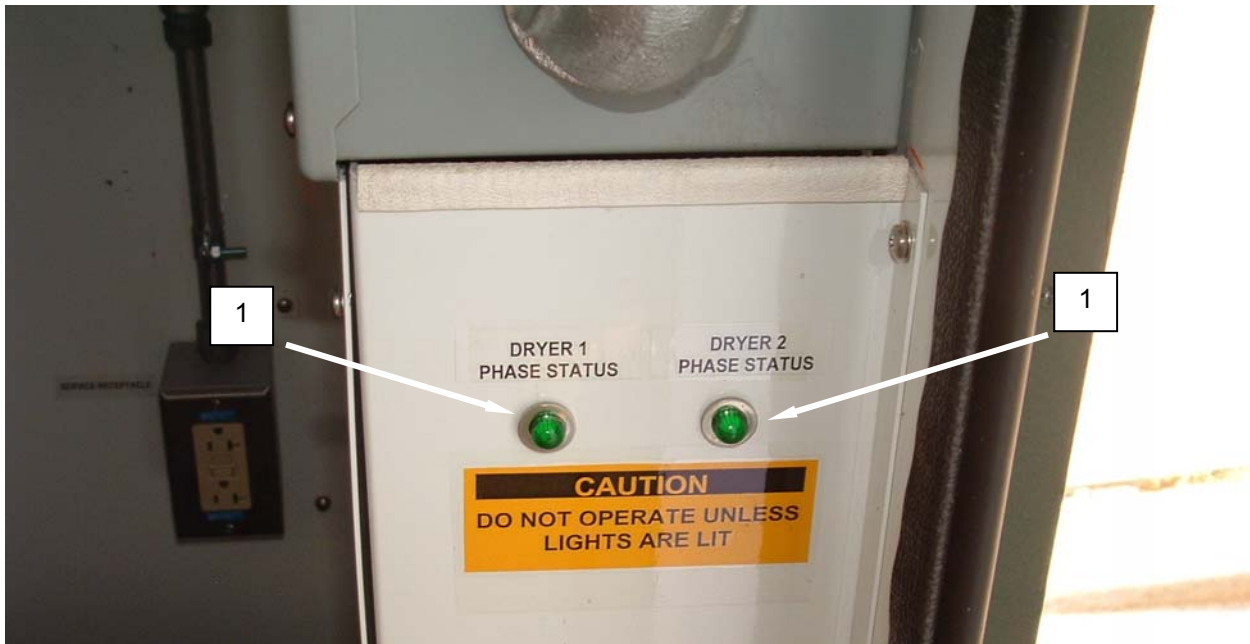
Figure 1. Phase Sequence Indicator Lights.
