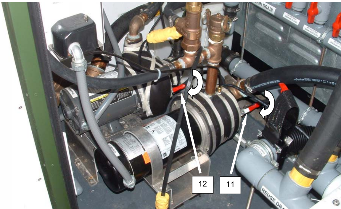
Figure 6. Drain Valves.
