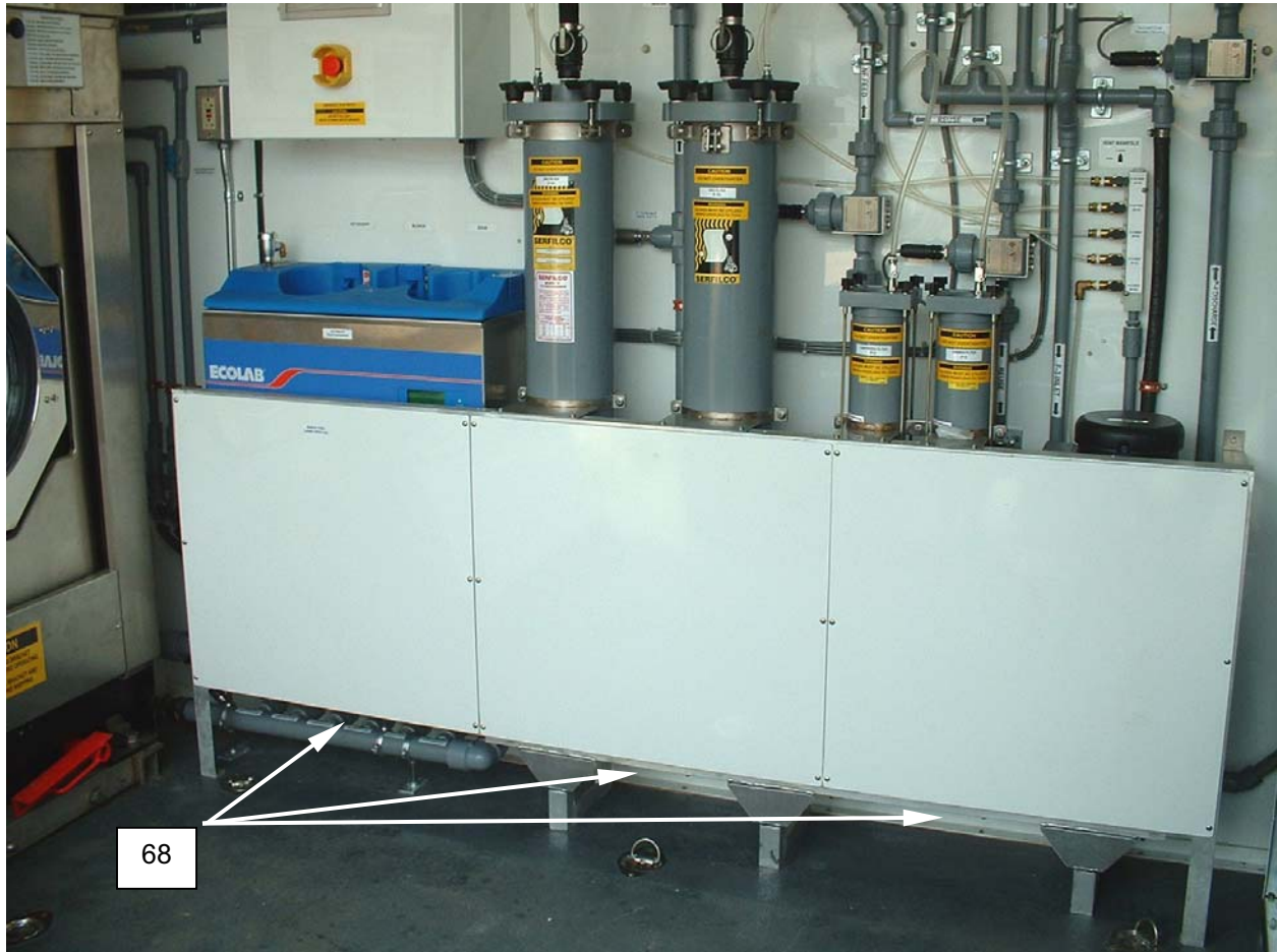
Figure 35. Install Panels.
