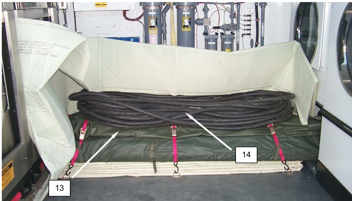
Figure 11. Placing the Cable.
