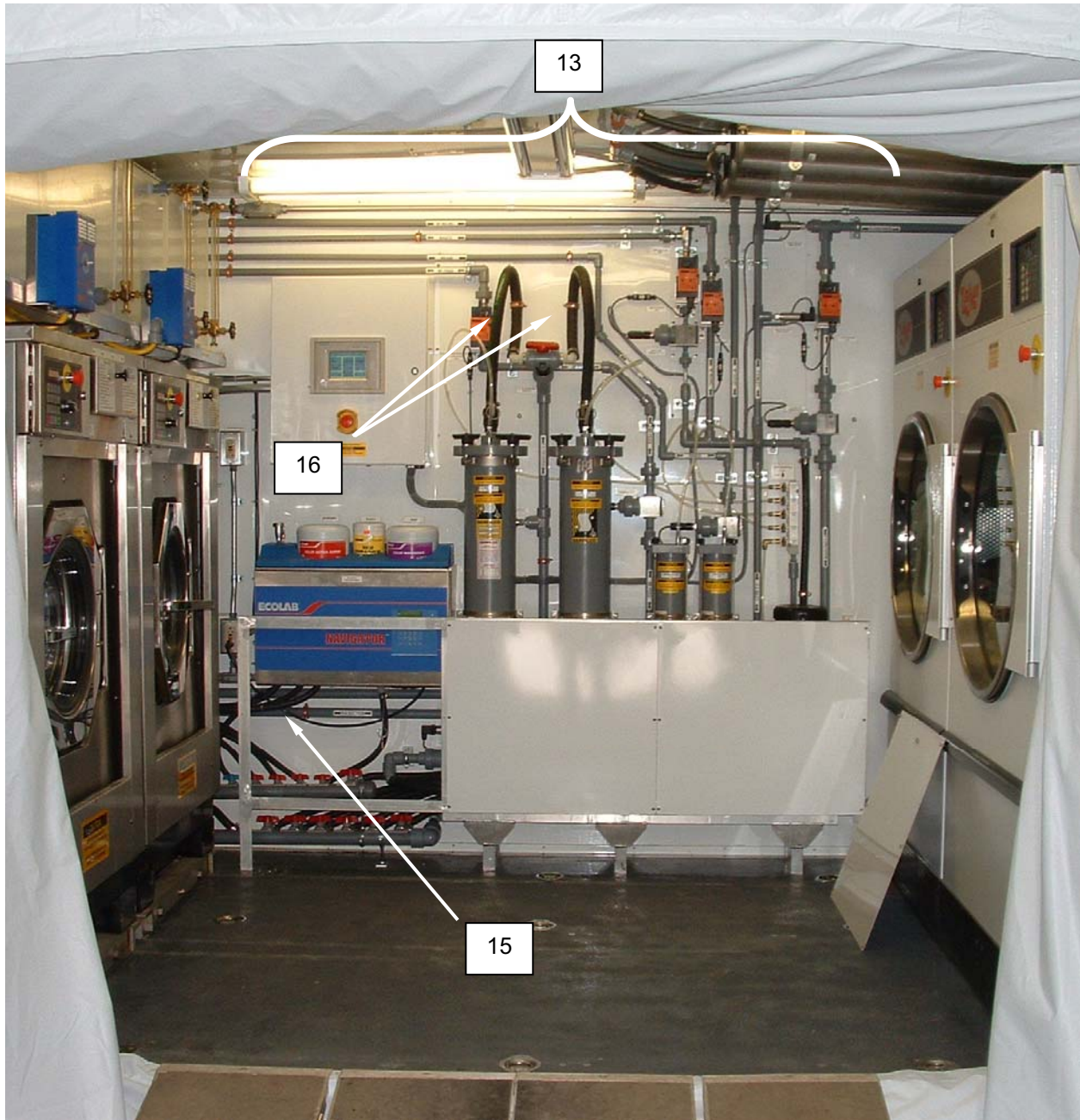
Figure 4. Before PMCS for Plumbing.
