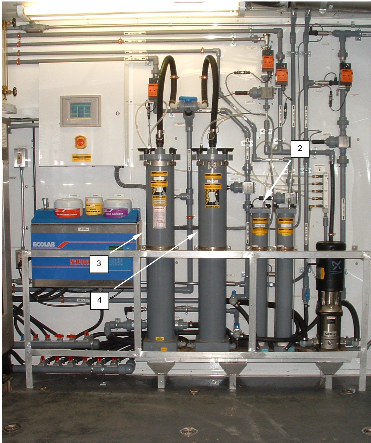
Figure 9. F2 Micron Differential Pressure High Alarm on PLC Display.
