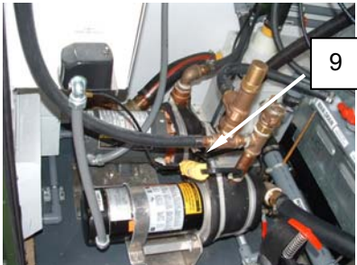
Figure 5. Operation in Severe Cold Conditions – Connect Heat Traces.
