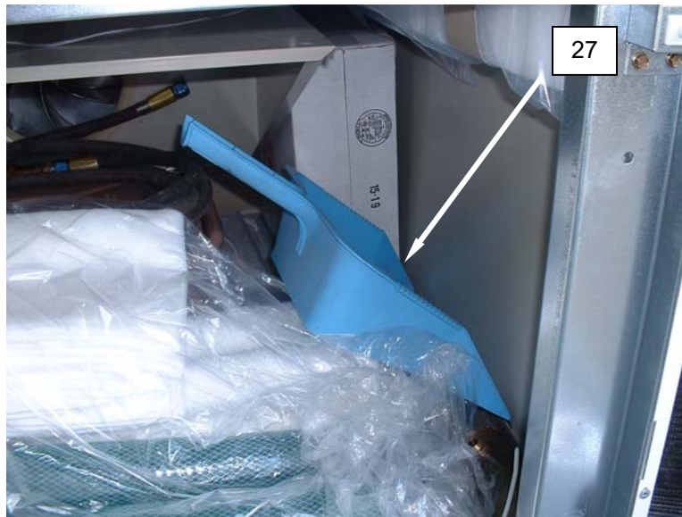
Figure 22. Dustpan between the Filters and the Dryer Cabinet.
