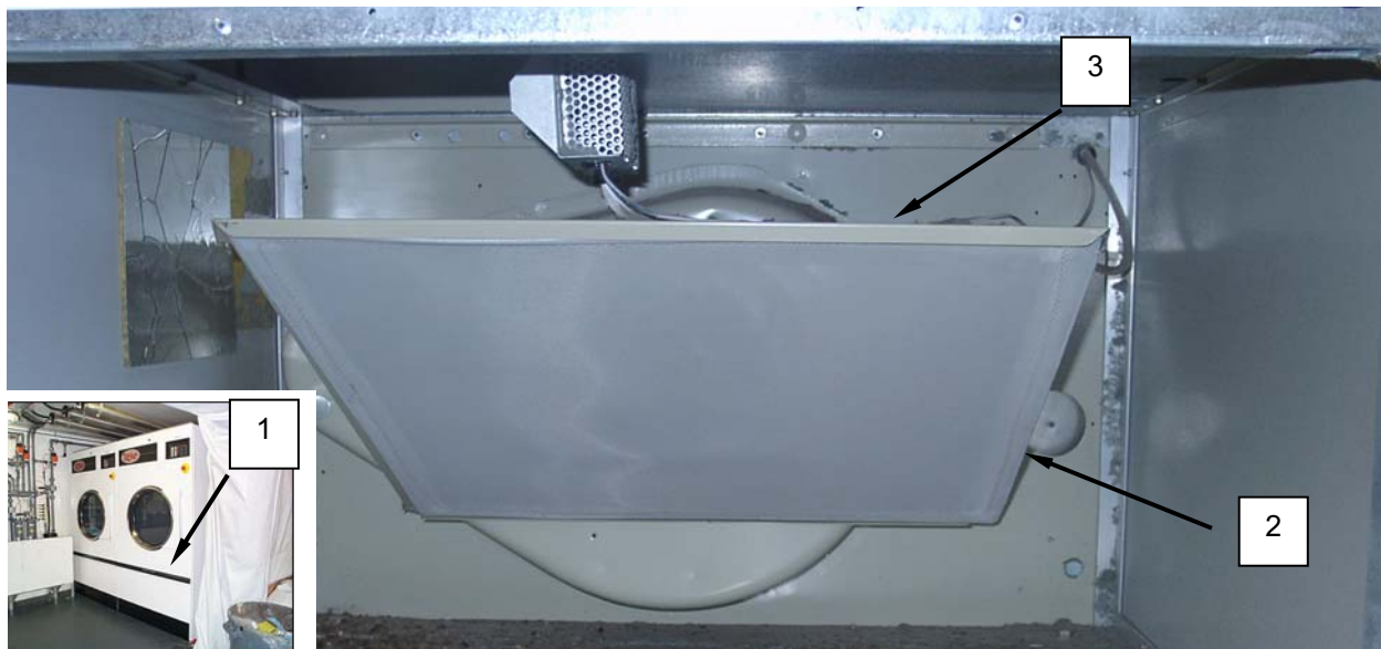
Figure 1. Clean the Dryer Lint Screen.
