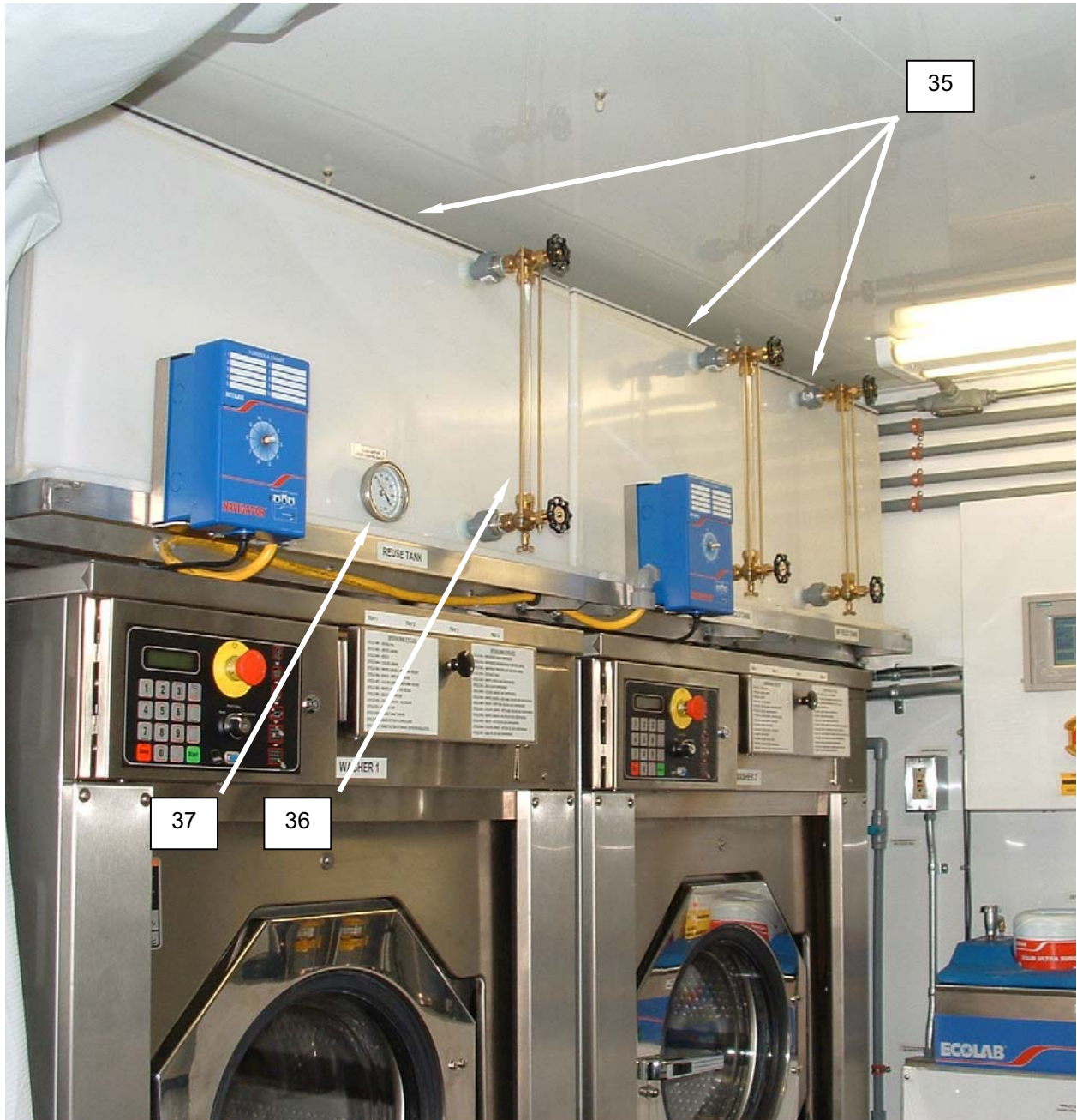
Figure 12. Before PMCS – Water Treatment System Holding Tanks.
