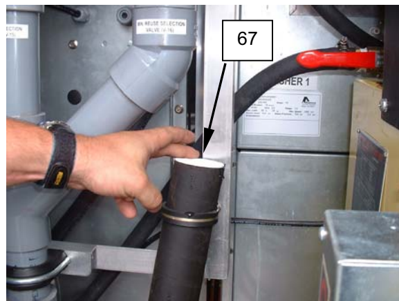
Figure 34. Add Antifreeze - Waste Water Tank.
