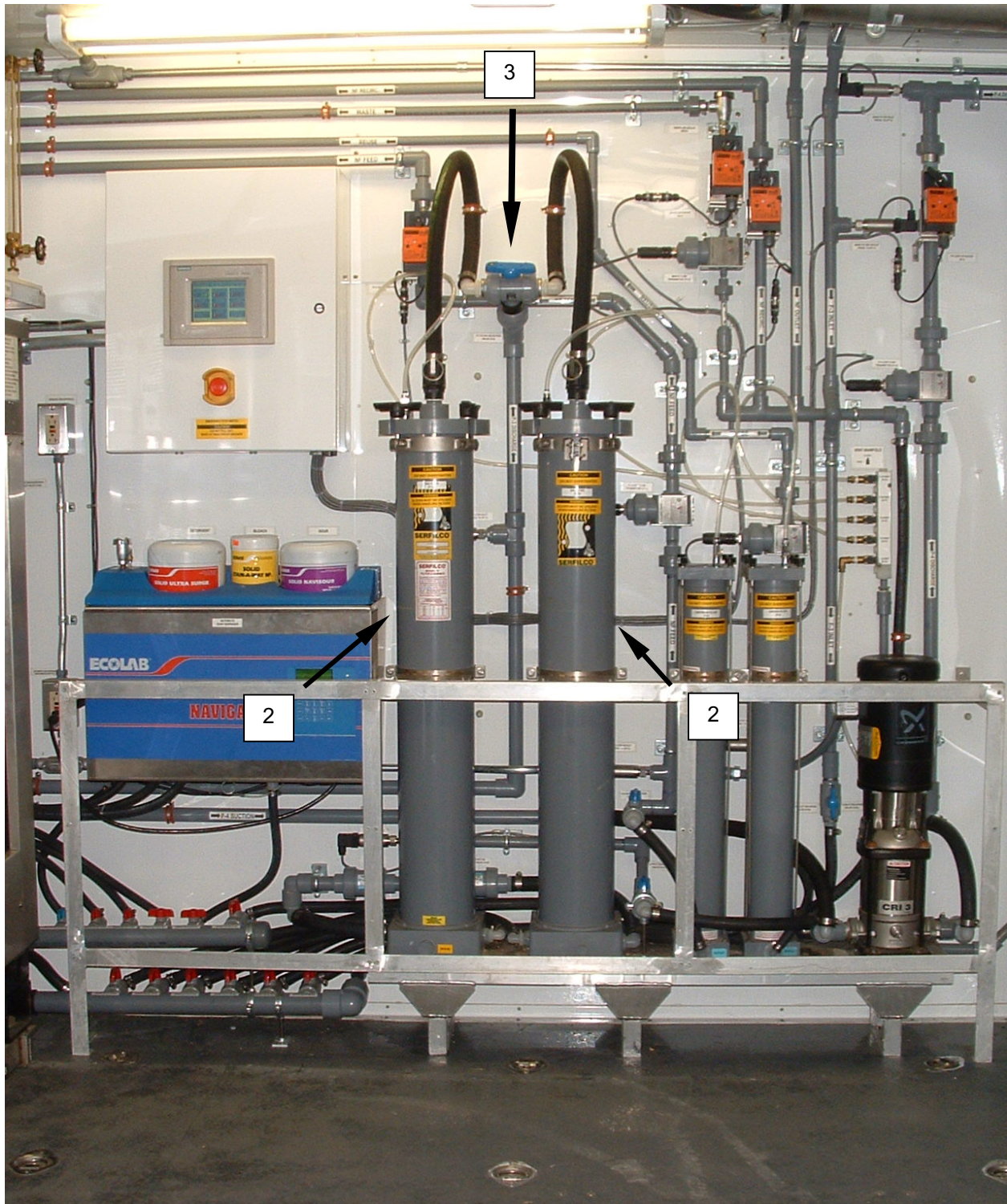
Figure 7. F1 Bag Filter is Clogged – P3 Pump is Stopped Alarm on PLC Display.
