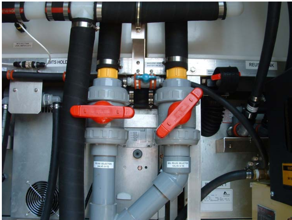
Figure 5. Valve Setting for Minimum Water Reuse.
